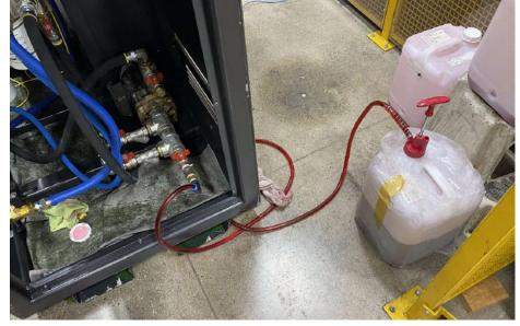
6. Open/Close ball valves based on images above to allow oil flow.
