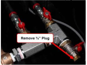
2. Place ball valves shown below in the required open or closed position
